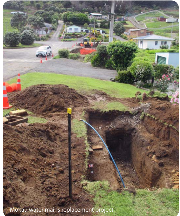
Mokau water mains replacement project
